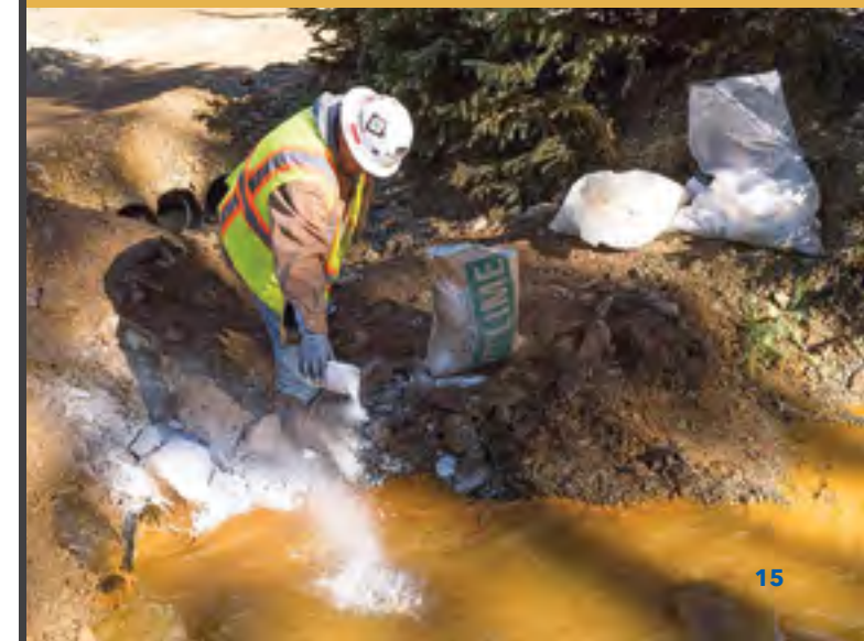
Below: Lime is added to a settling pond to assist in the pH adjustment of the water prior to discharge to Cement Creek on August 14th, 2015. Photos: Eric Vance / EPA
